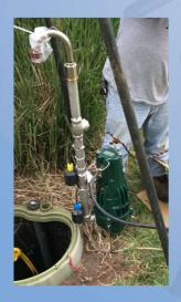
Non-Contact switches require an unobstructed path between the sewage and the switch. Non-Contact switches by nature are not submersible. When utilizing "air capture" type columns or chambers, the likelihood for grease obstruction is high. Non-contact switches are intended to operate in a dry environment; locating them inside a wet well or relying upon atmospheric pressure equalizing chambers (full of humid air) can be problematic. Cleaning usually requires skilled disassembly and reassembly.
